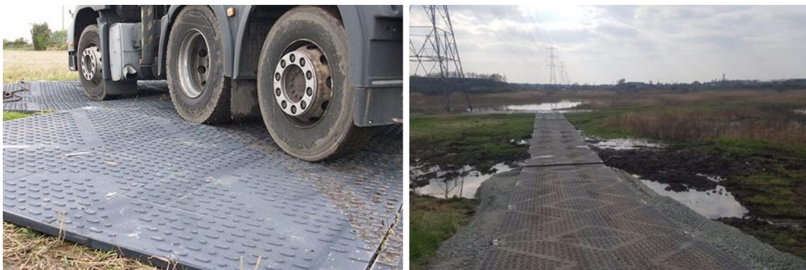
Figure 6-2 Examples of track mats 1
