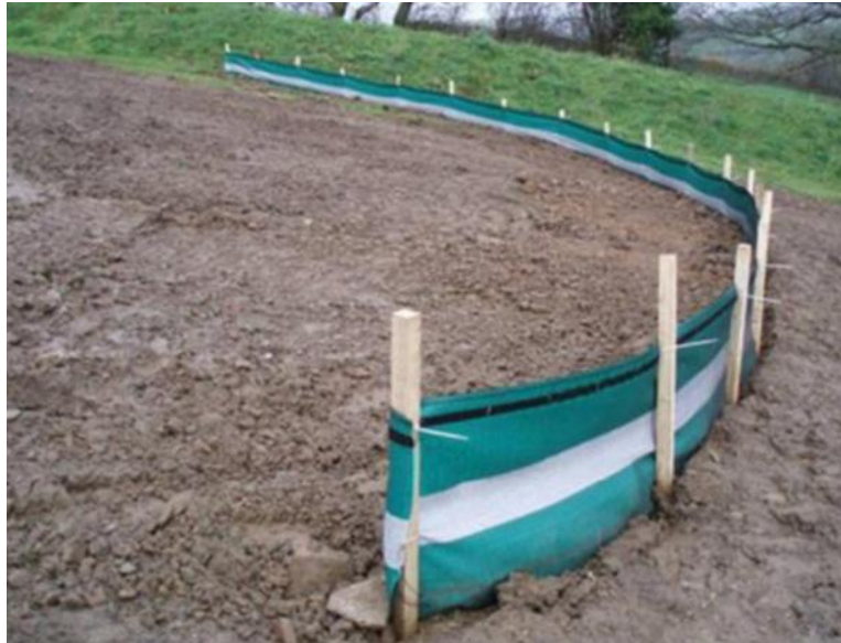
Figure 6-1: Example of suitable silt fence mitigation ensuring maximum safeguarding efficiency.
